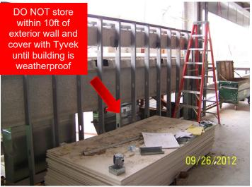
According to the manufacturer(s) and GA-801, the delivered product must be stored in a protected area from direct sunlight exposure, fully protected from weather, and avoid condensation.
